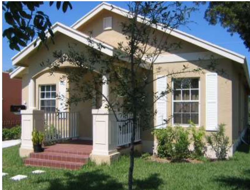
Typical CLT home in Northwood
